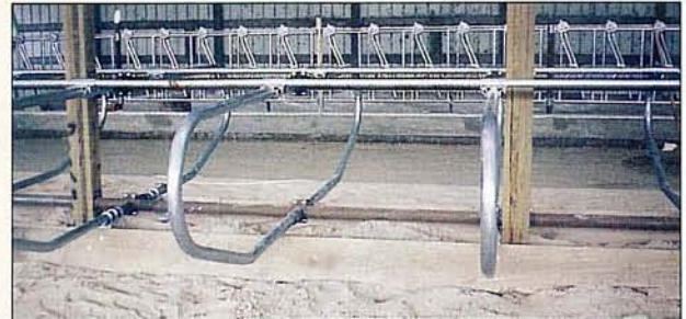
INFRASTRUCTURE shown with ALBERS cantilever freestall loops installed.
